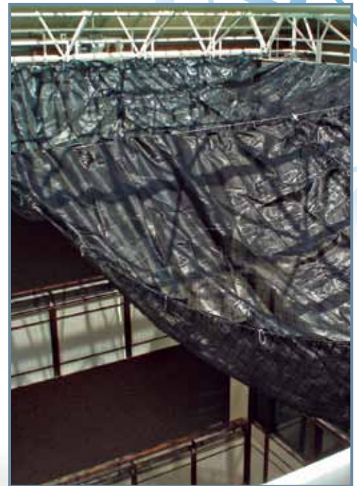
Aetna Atrium Renovation, Hartford, CT
