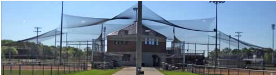
Overhead Bleacher and Concession Protection
