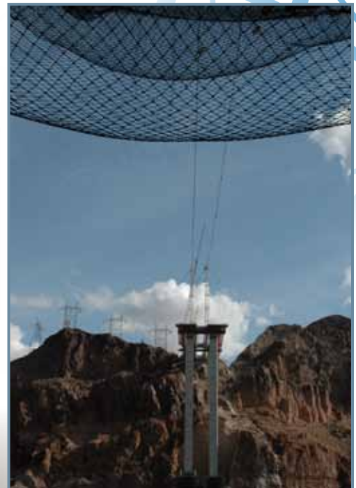
Hoover Dam Bypass Project US 93
